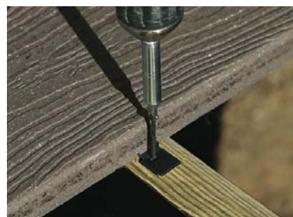
Hidden Fastener Installation to Joist
