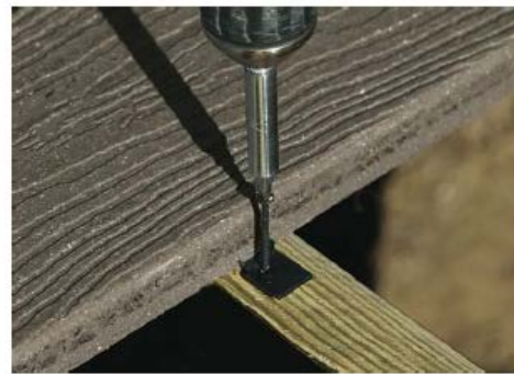
Hidden Fastener Installation to Joist
