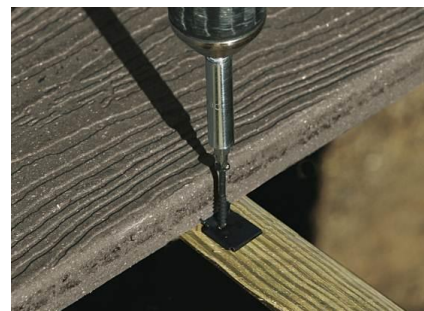
Hidden Fastener Installation to Joist
