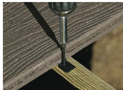
Hidden Fastener Installation to Joist
